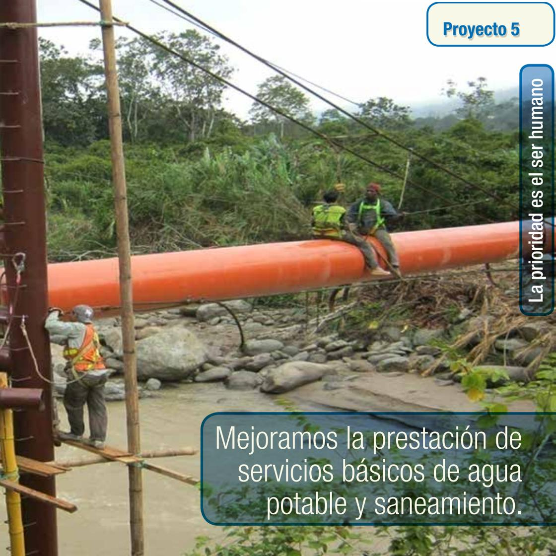
A photograph showing a construction site in a rural, hilly area. A large, bright orange pipe is being laid across a river. Two workers are sitting on the pipe, while another worker stands on a wooden platform near a metal structure on the left. The background features lush green vegetation and a rocky riverbed.
